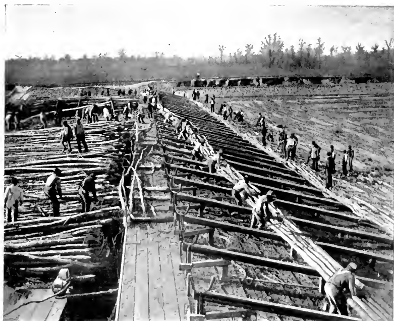
CONSTRUCTING FASCINE MAT ON MATTRESS WAYS.
